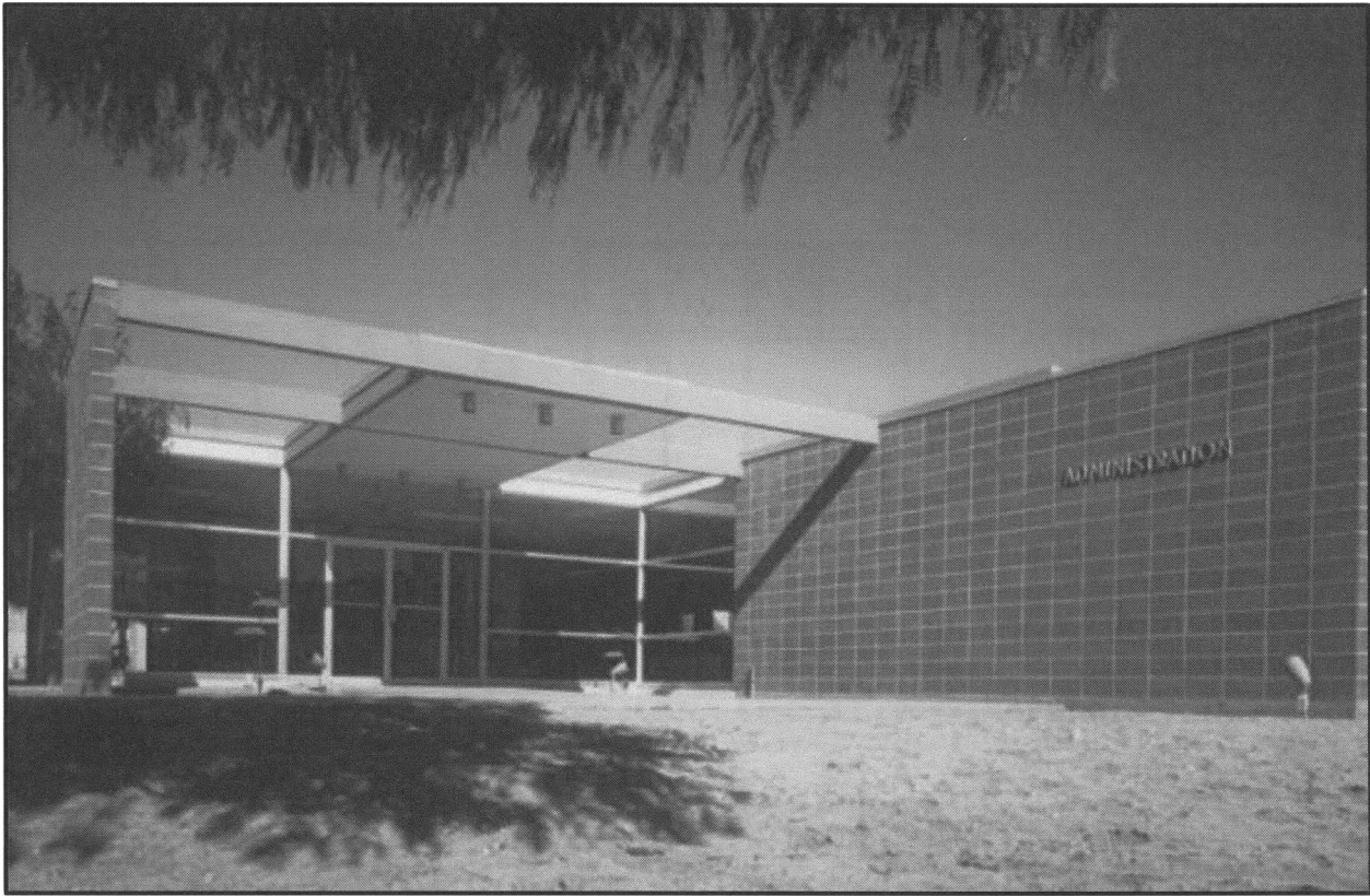
Photograph 5: Administration Building, front entrance, 1957-58. (Photograph courtesy of Donald Wexler Collection, ENV Archives Special Collections, Cal Poly Pomona)
