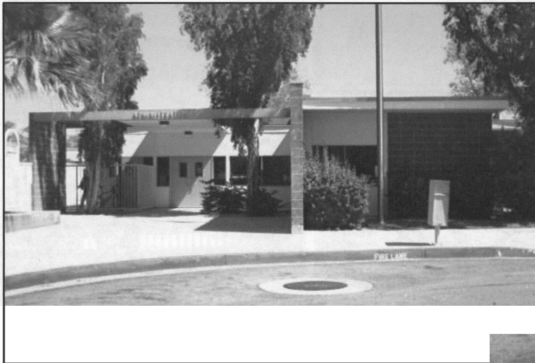
Photograph 8: Front entrance to building after alterations of 2000. View looking north.
