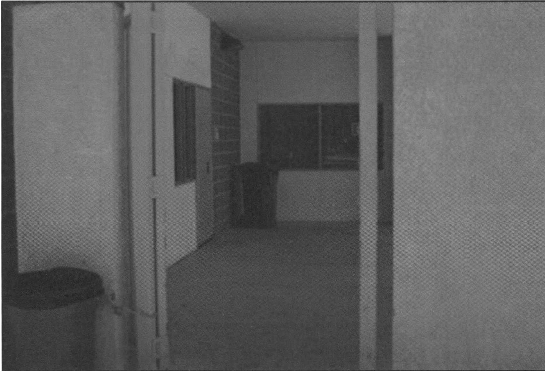
Photograph 9: View of north wall of the original lobby space after alterations of 2000. A glass curtain wall with a set of full-length glass doors had been situated here to open the lobby space to a view of the north lawn area.
