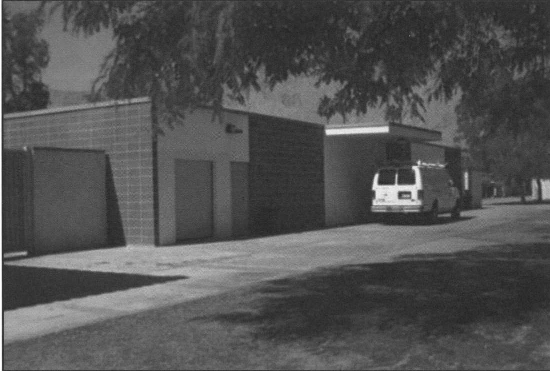
Photograph 11: North elevation of building showing the awning and solid infill wall where there originally was an open patio area for the building. View looking southwest.
